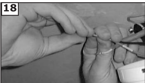
18 Make wire connections to power source using wire nuts provided. Make sure that no filiments are outside of the wirenut. After making the wire connections, the wires should be spread apart with the grounded conductor and the equipment-grounding conductor on one side of the outlet box and ungrounded conductor on the other side of the outlet box. The splices after being made should be turned upward and pushed carefully up into the outlet box.
